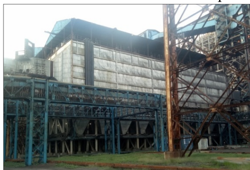
Fig 2: Electro Static Precipitator at NTECL
