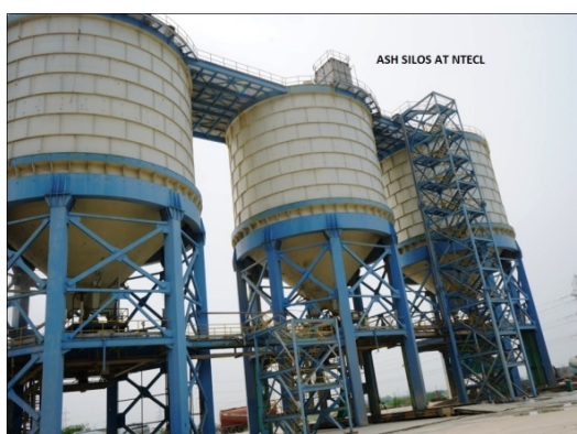
Fig 5: 3 No of Dry ash silos at NTECL
