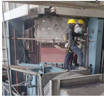
Fig 4: NO x reduction – combustion modification works in boiler
